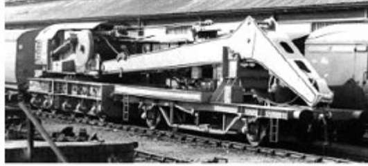
V Steam Driven Crane
